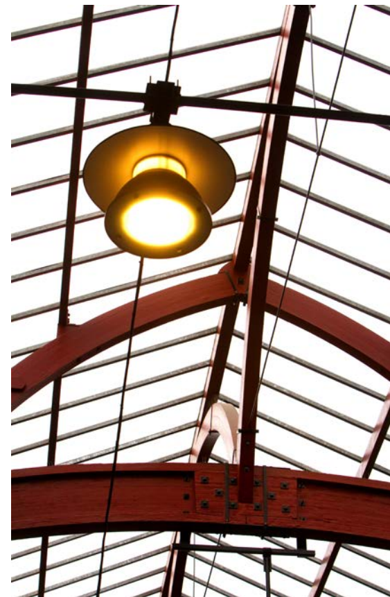
Malmö Central Railway Station, Sweden.
