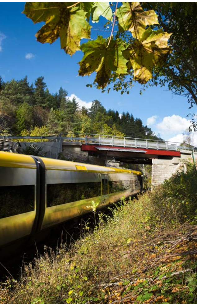
Railway bridge, Munkedal, Sweden.
