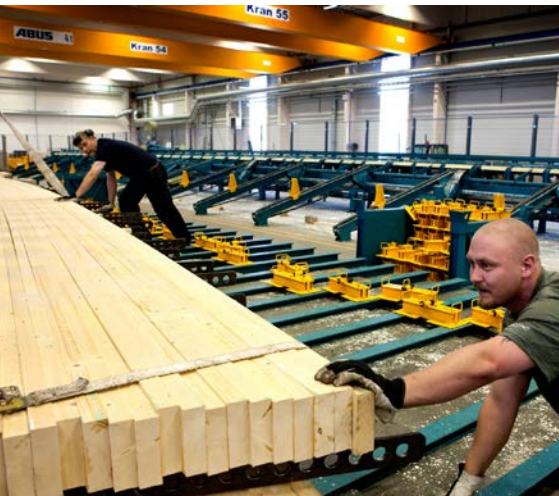
Manufacture of curved glulam elements.
