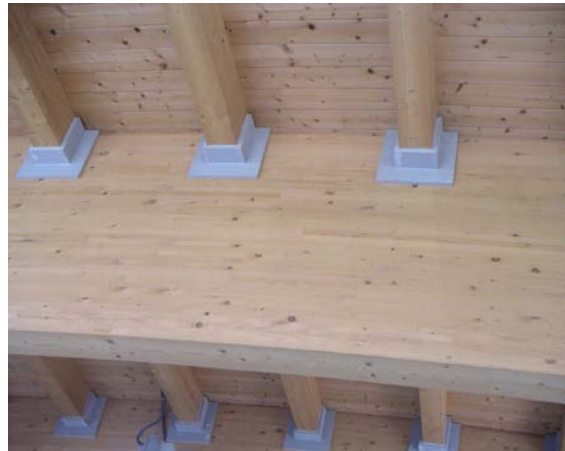
Figure 16.16 Protection of end-pin-support by means of asbestos-free calcium silicate plates
