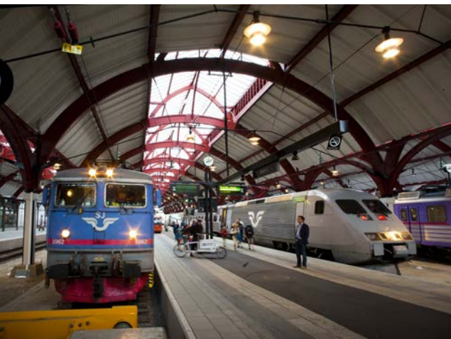
Malmö Central Railway Station, Sweden.
