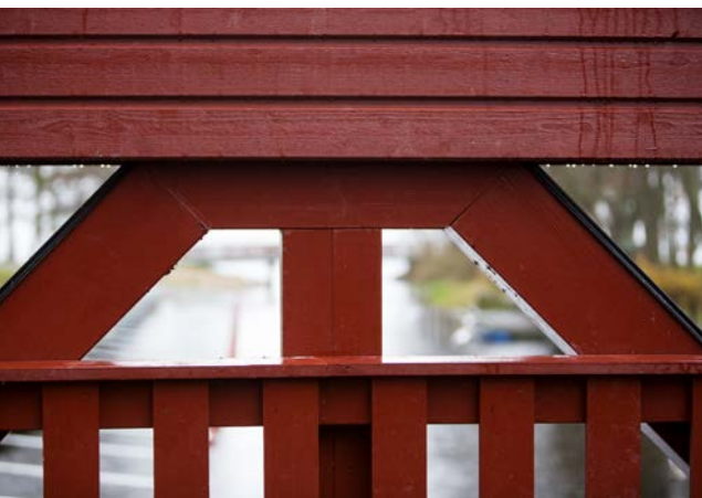
Bridge, Ringsjöstrand, Sweden.
