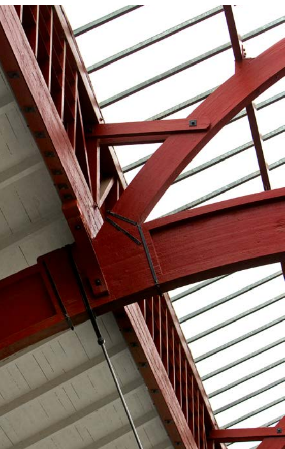
Malmö Central Railway Station, Sweden.
