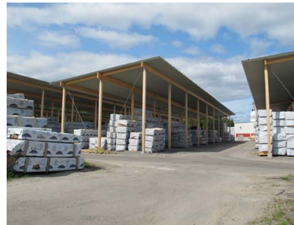
Timber warehouse, Sundsvall.
